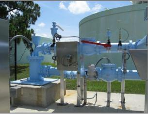
Photo 3-2. (L) City of Sanford, FL ASR Well; (R) City of Sanford, FL ASR Wellhead
