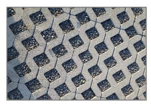
Photo A4-2. Example of Permeable Pavement
